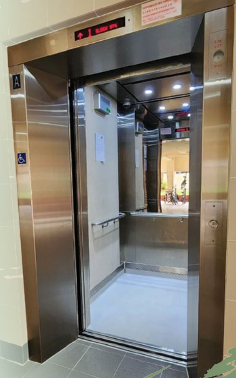
Lift Replaced at Pasir Ris Blk 576
